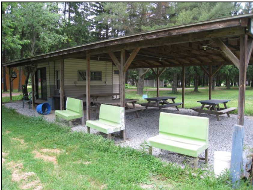
GAMES BUILDING AND SHELTER
